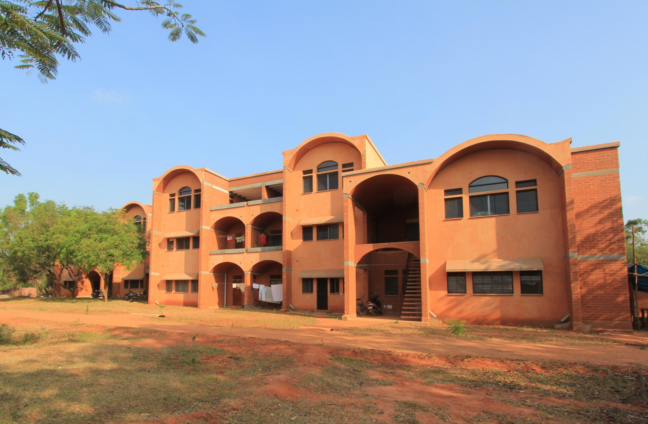
Realization housing, Auroville - 8 Apartments completed in 2011
