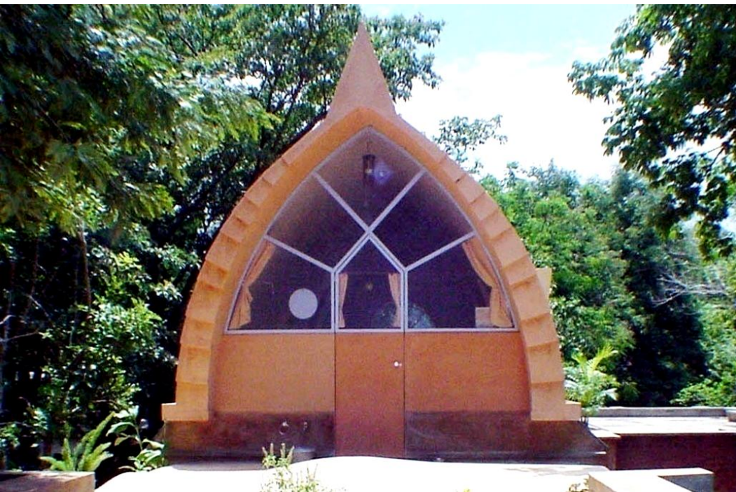
House at the Auroville Earth Institute, built with the Free Spanning Technique
