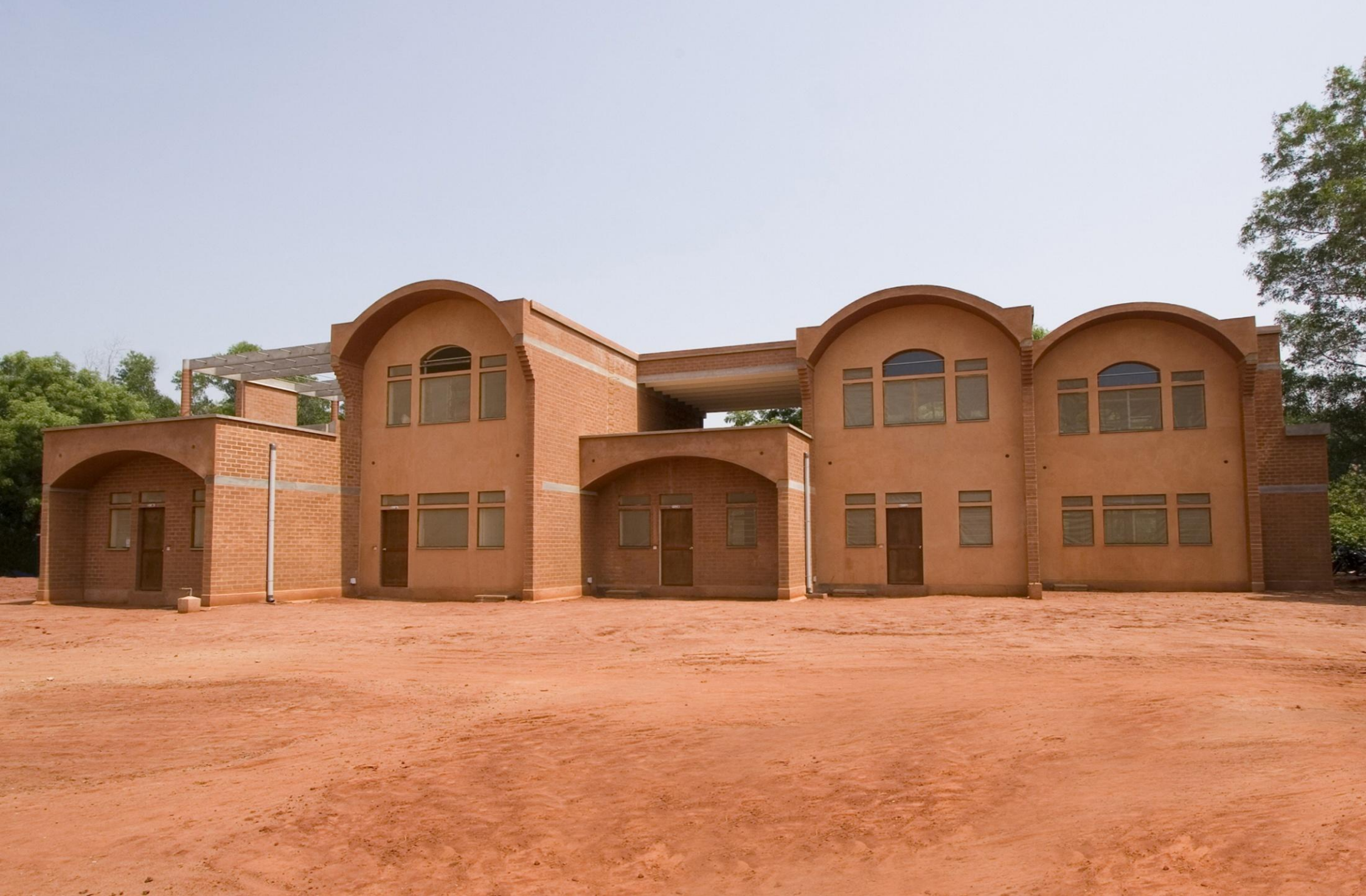
Realization housing, Auroville - 5 Apartments completed in 2010
