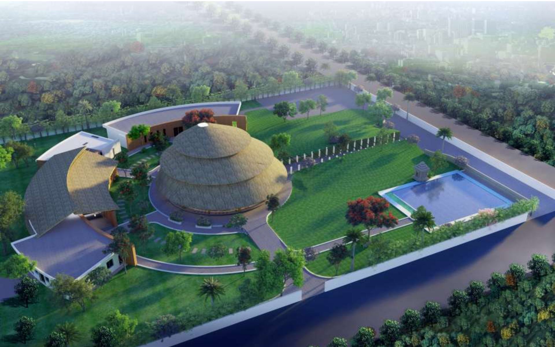
OVERALL AERIAL VIEW
