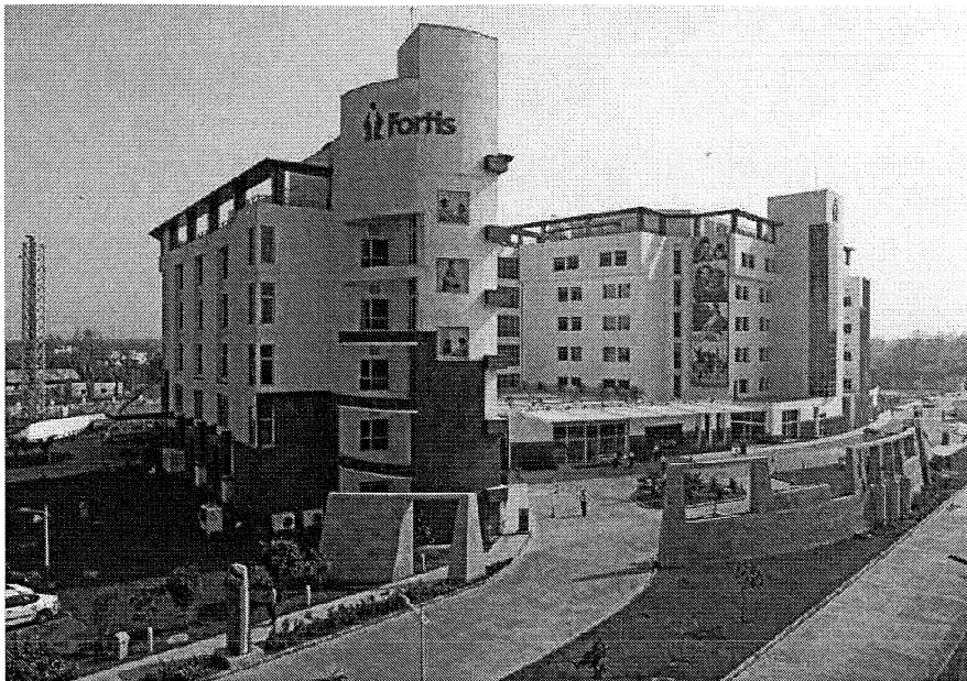
Figure 2: FORTIS Shalimar Bagh, 3-star TERI-GRIHA rated (provisional rating).
