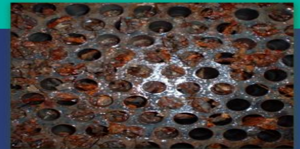
Fouled Condenser Tubes
