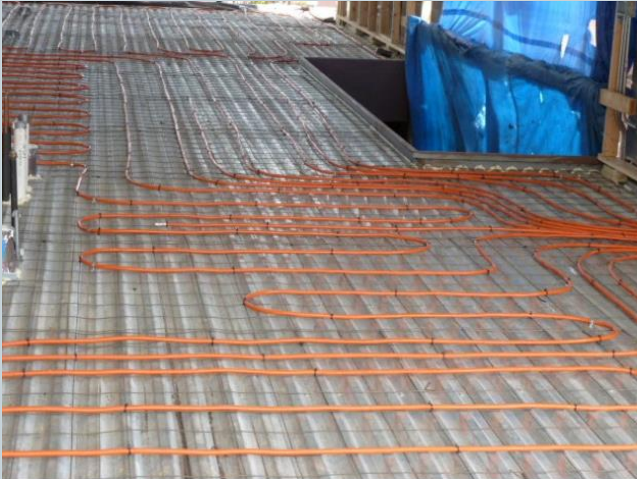
Radiant Tubing in floor
