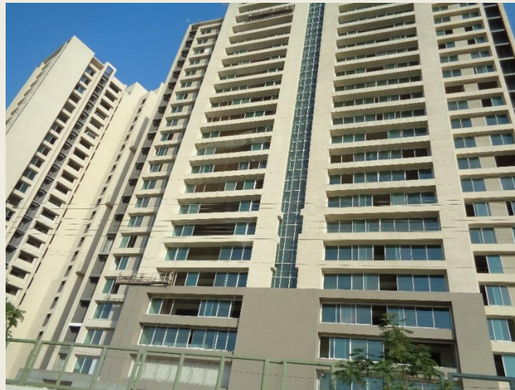
WWR \sim 35\% Inadequate Shading of Windows
