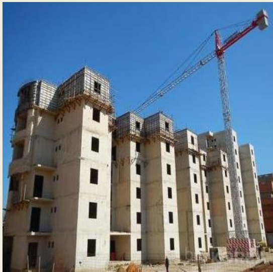
U (wall) \sim 3.5 \text{ W/m}^2.\text{K} Monolithic concrete wall
