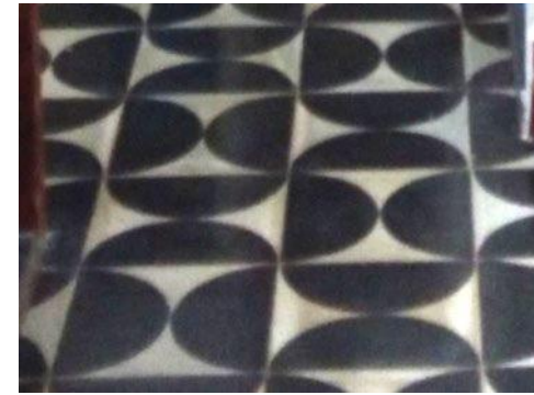
'Atthangudi' Tiles manufactured at site
