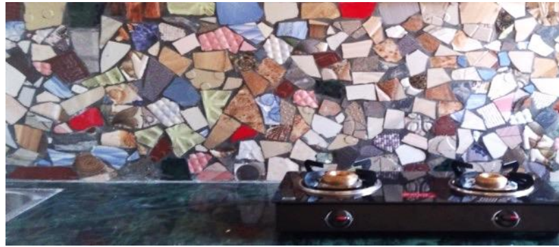
Broken Vitrified Tiles Terrazzo mosaic for Dado
