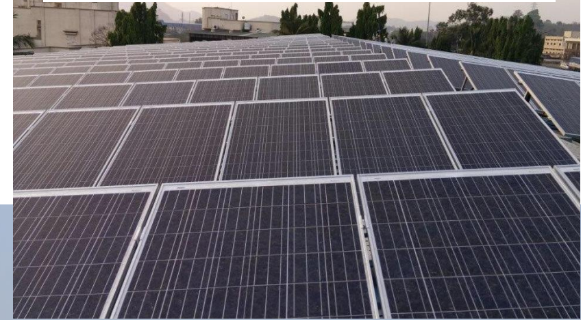
Pitched roof; non-penetrating
