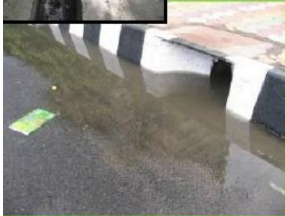
Overflowing Storm Water Inlet, ITO
