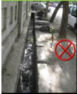
Silted Open Drain, Tughlaqabad Institutional Area
