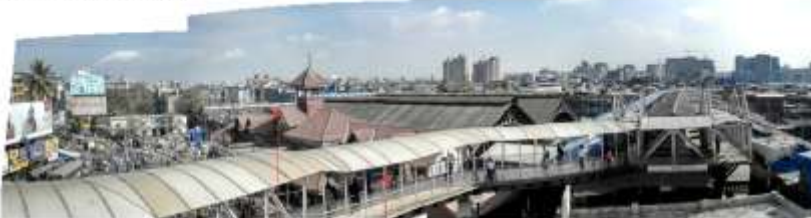
EXISTING RAILWAY STATION : BANDRA RAILWAY STATION
