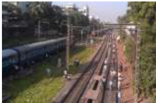
Existing Train Tracks & Elevated Pipe Lines
