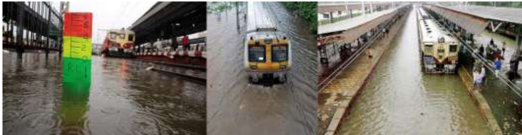
High tide + torrential rain + poor drainage
