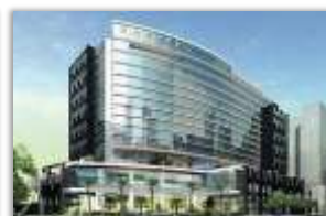
The 5 Star Sofitel Hotel, Mumbai HVAC, Electrical, Plumbing, Fire fighting
