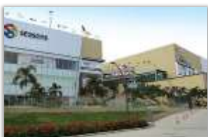
Seasons Mall, Magarpatta HVAC & Fire Fighting
