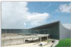
Netaji Subhash Chandra Bose International Airport, Kolkata HVAC, Electrical works, Plumbing, Water treatment
