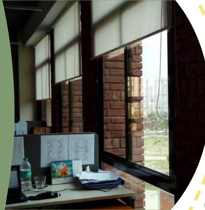
Image showing vertical fins for shading windows & natural light in the office space.
